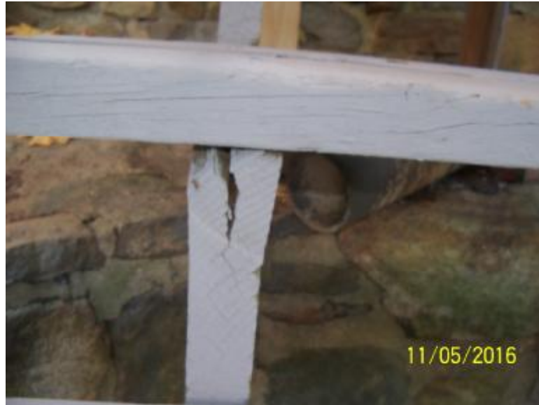
Figure 6. Split stringer where the tread is nailed.
