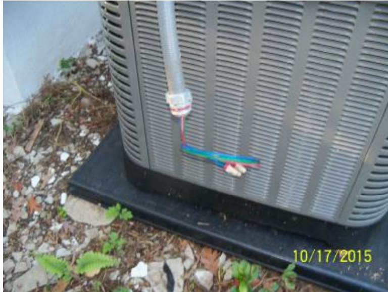
Figure 10. Cable is not connected to the AC unit.
