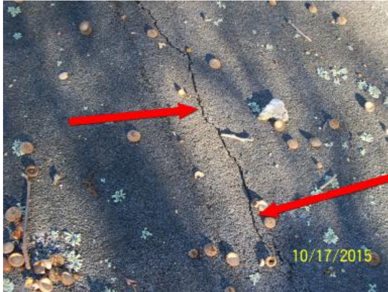
Figure 4. Cracked rolled roof material.
