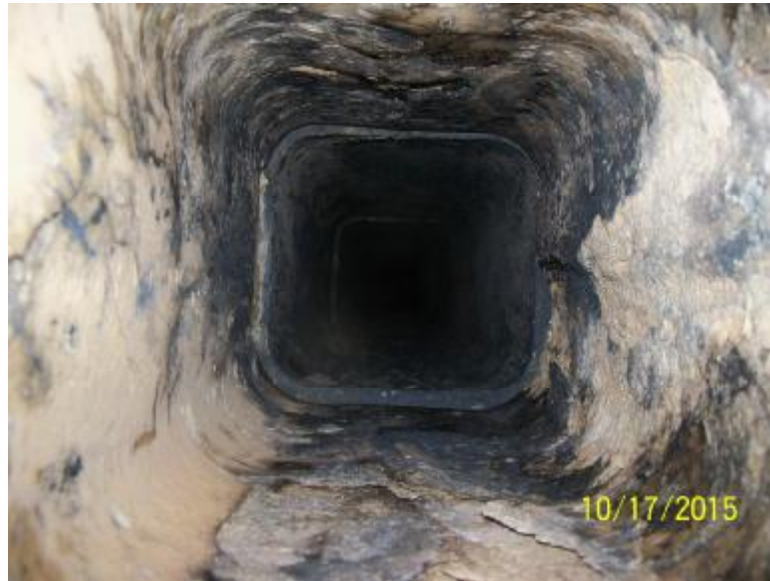
Figure 5. Deteriorated liner.
