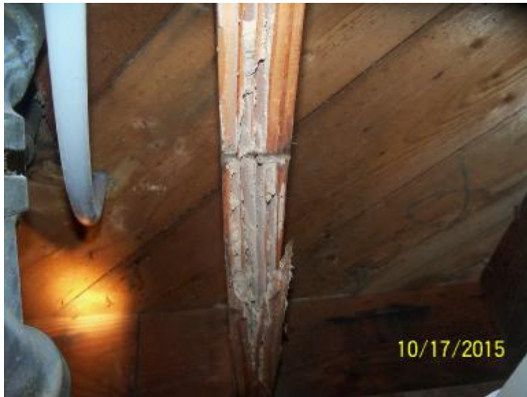
Figure 7. Termite damaged joist. See section 1607 below.
