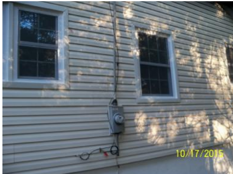
Figure 1. Overhead electrical service cables are too close to operable windows. See section 1110 below.
