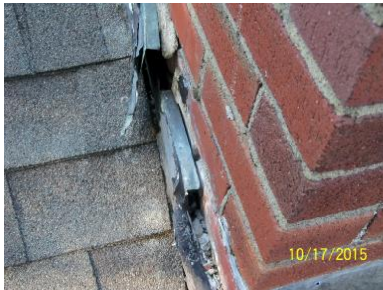
Figure 3. Large gaps, loose flashing at chimney.
