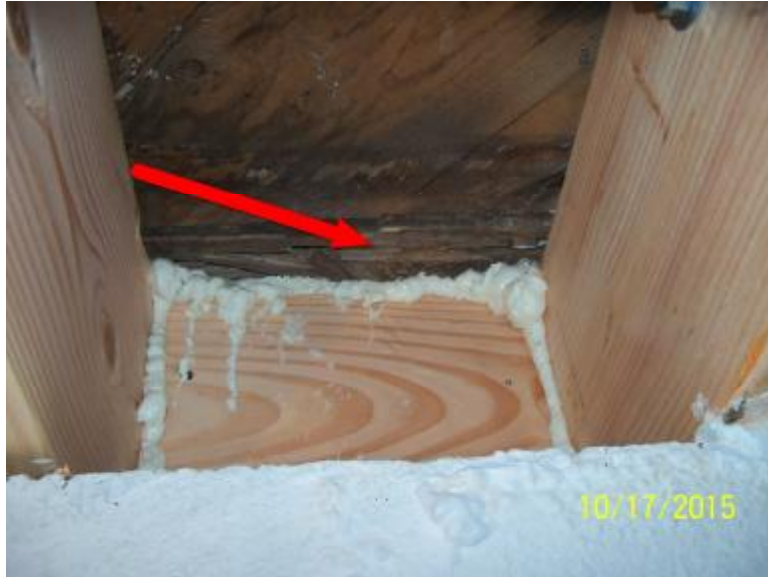
Figure 8. Front section of house, under the main entry. Note the water damaged wood that was covered with new wood.
