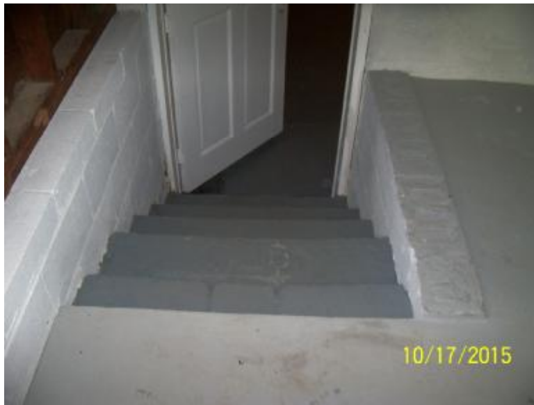
Figure 6. Missing hand and guardrails.
