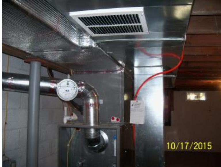
Figure 9. Return air grill within 10 feet of the barometric damper.
