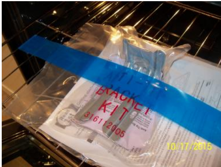
Figure 12. The anti-tip bracket was left inside the oven.
